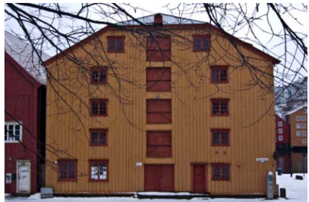
Warehouse on the waterfront.
